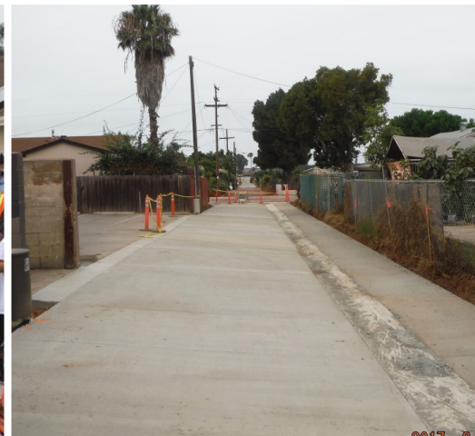
Green infrastructure projects, such as green alleys, have water quality benefits including retention and infiltration of storm water and removal of trash, sediment, and nutrients
