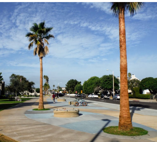
The Elm Avenue Street Improvement project reduces storm water runoff while providing significant pedestrian, biking, and traffic calming improvements.
