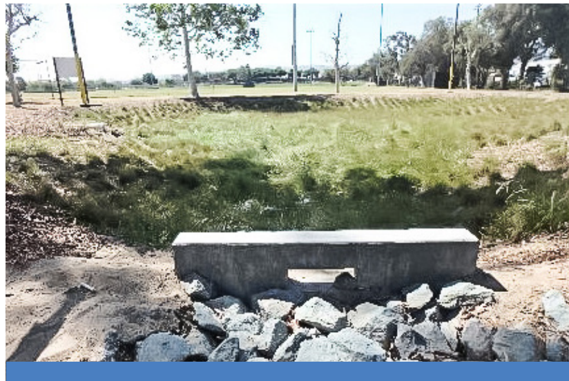
The City of San Diego constructed green infrastructure at the Cesar Chavez Community Center to treat runoff from 3.31 acres and meet the 2018 alternate interim goal.
