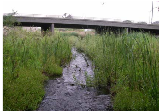
Figure ES8-7. Los Peñasquitos Creek Highway 805 Site.
