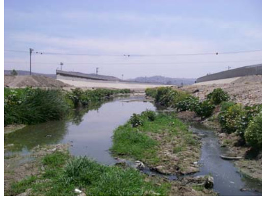
Figure ES12-7. Border Fence Site
