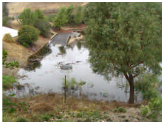
Stowe Drive SUSMP Basin during treatment of storm water
