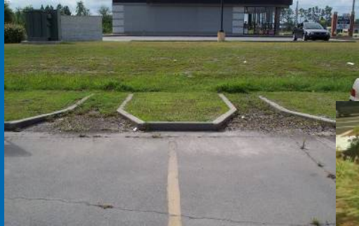
Parking lot drains to swale
