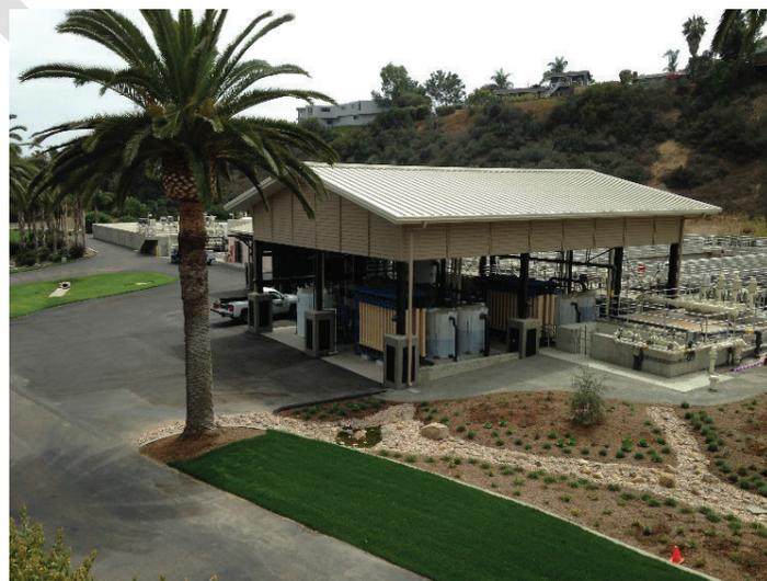
distribute up to 2.48 million gallons per day (MGD) of tertiary-treated wastewater to recycled water users. It is also permitted to discharge up to 5.25 MGD of secondary-treated wastewater to the Pacific Ocean through the San Elijo Ocean Outfall, 1.5 miles offshore.
