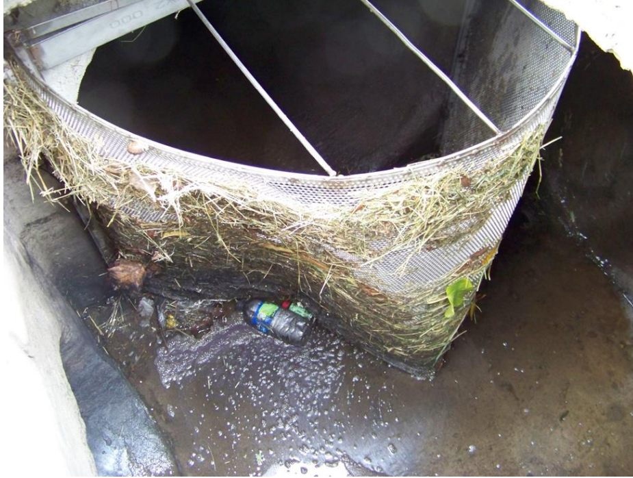
FIGURE J- 3. EXAMPLE OF A FULL CAPTURE DEVICE WITH A CLOGGED SCREEN
