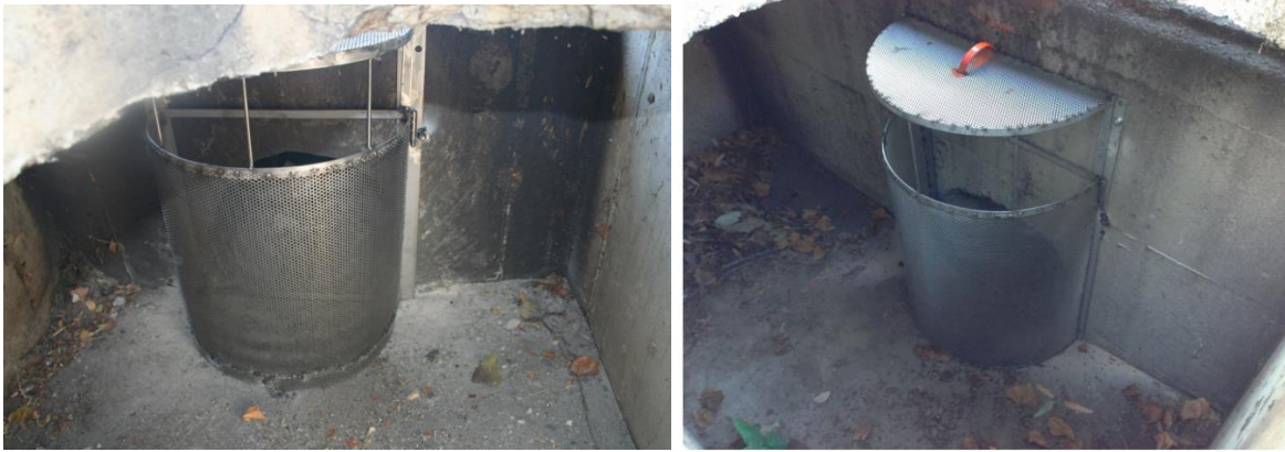
FIGURE 1. EXAMPLE OF INSTALLED STORMTEK CONNECTOR PIPE SCREEN FULL CAPTURE DEVICE
