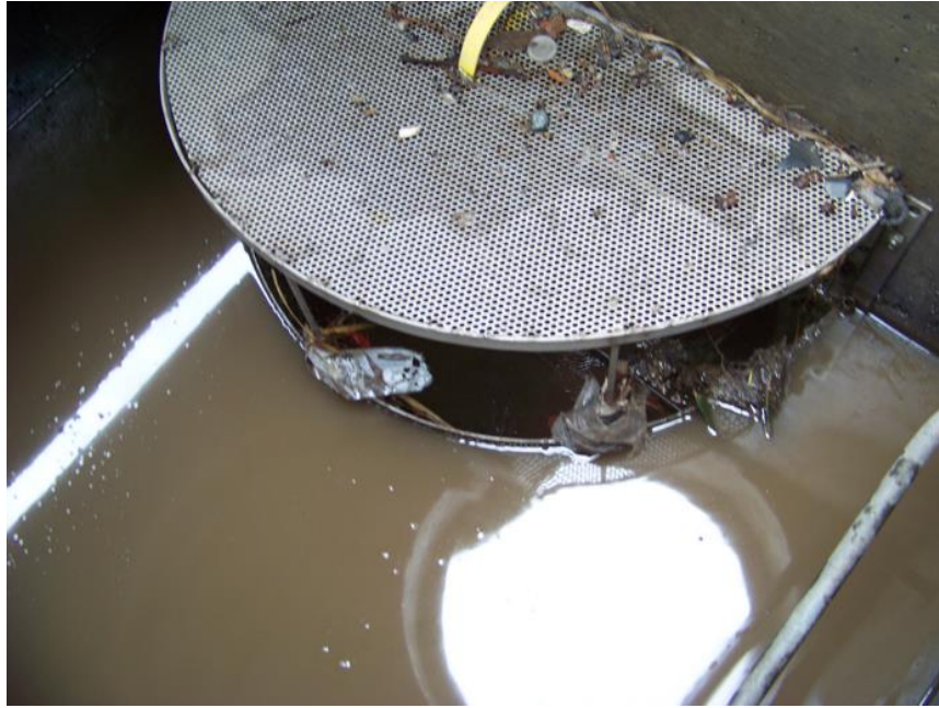
FIGURE J- 1. EXAMPLE OF A FULL CAPTURE DEVICE WITH A CLOGGED SCREEN
