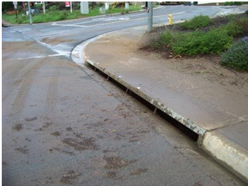
FIGURE J- 2. EXAMPLE OF FLOODING DUE TO A CLOGGED SCREEN OF A FULL CAPTURE DEVICE
